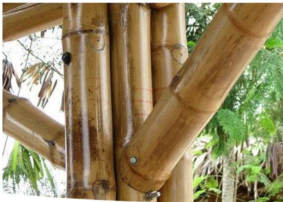
**Figure 20: Joinery used in the traditional bamboo houses**
