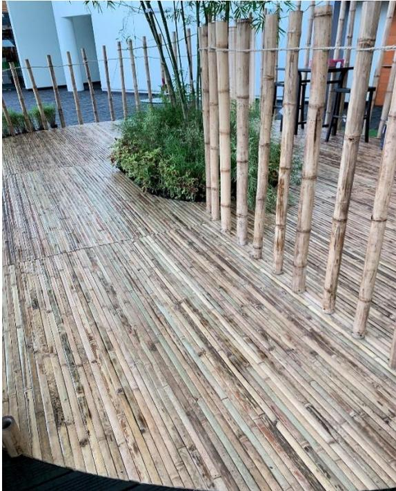
**Figure 18: Bamboo flooring from bamboo splits.**
